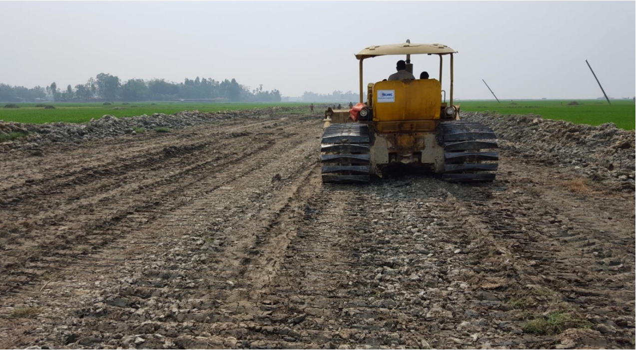
Grading of ROW Along Bibiyana-Dhanua 36" Diameter Pipeline
