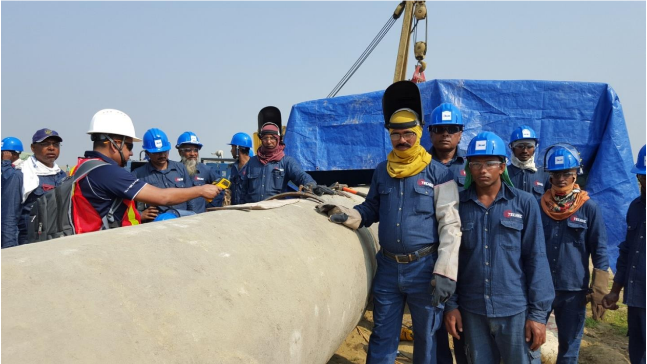
Preheat Test conducting by QA/QC Engineer
