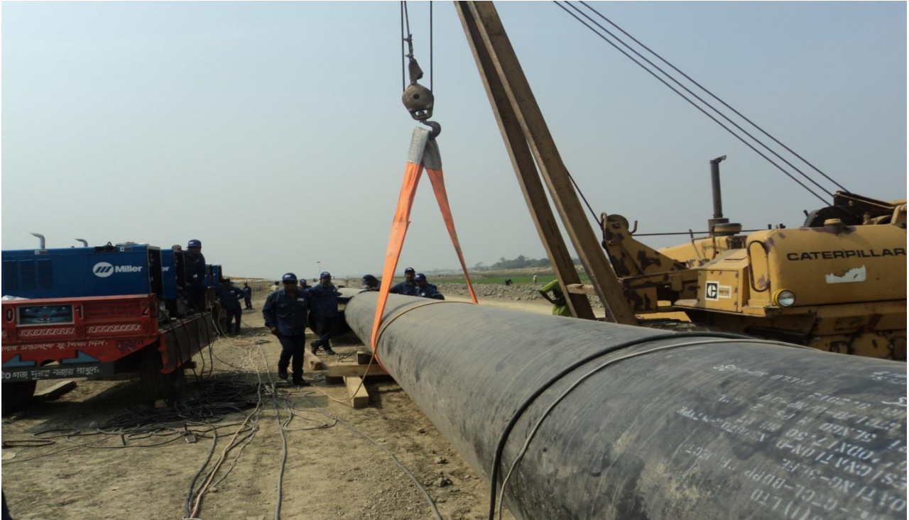
Natural Gas Transmission Line Production Welding
