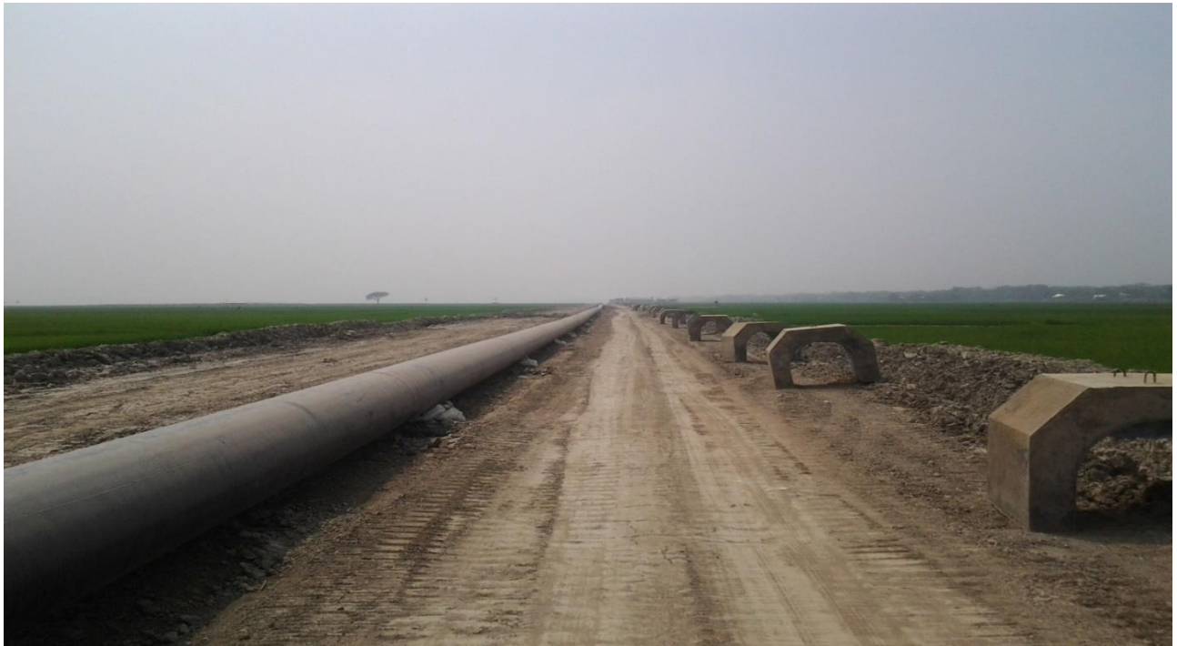
Constructed 36"Ø Pipeline are in waiting for
