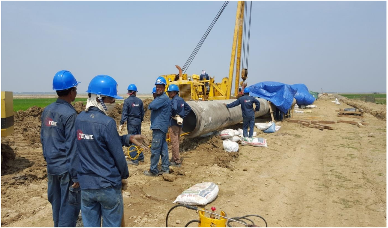
Aligning of 30"Ø Line Pipe for Fit up
