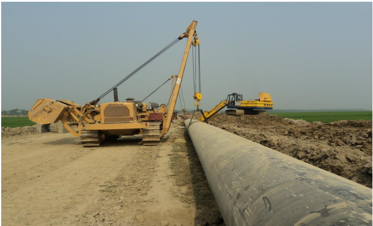
Trenching & Pipe Line Lowering
