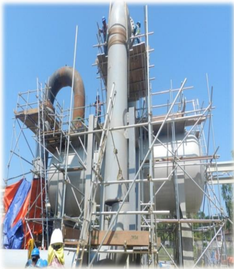
CLIENT: CHEVRON MECHANICAL & FABRICATION WELDING WORK AT MUCHAI COMPRESSOR
