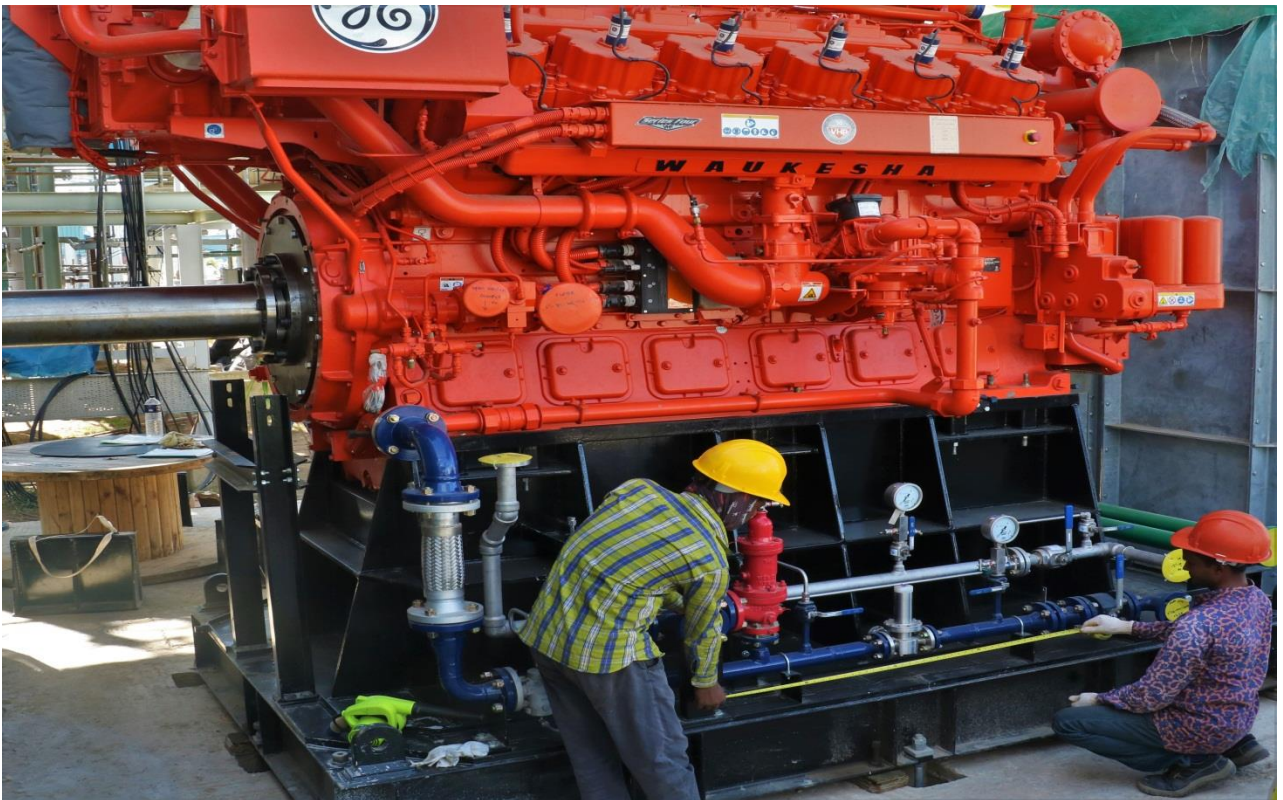
Equipment Installation in CRU Project, Hobiganj.
