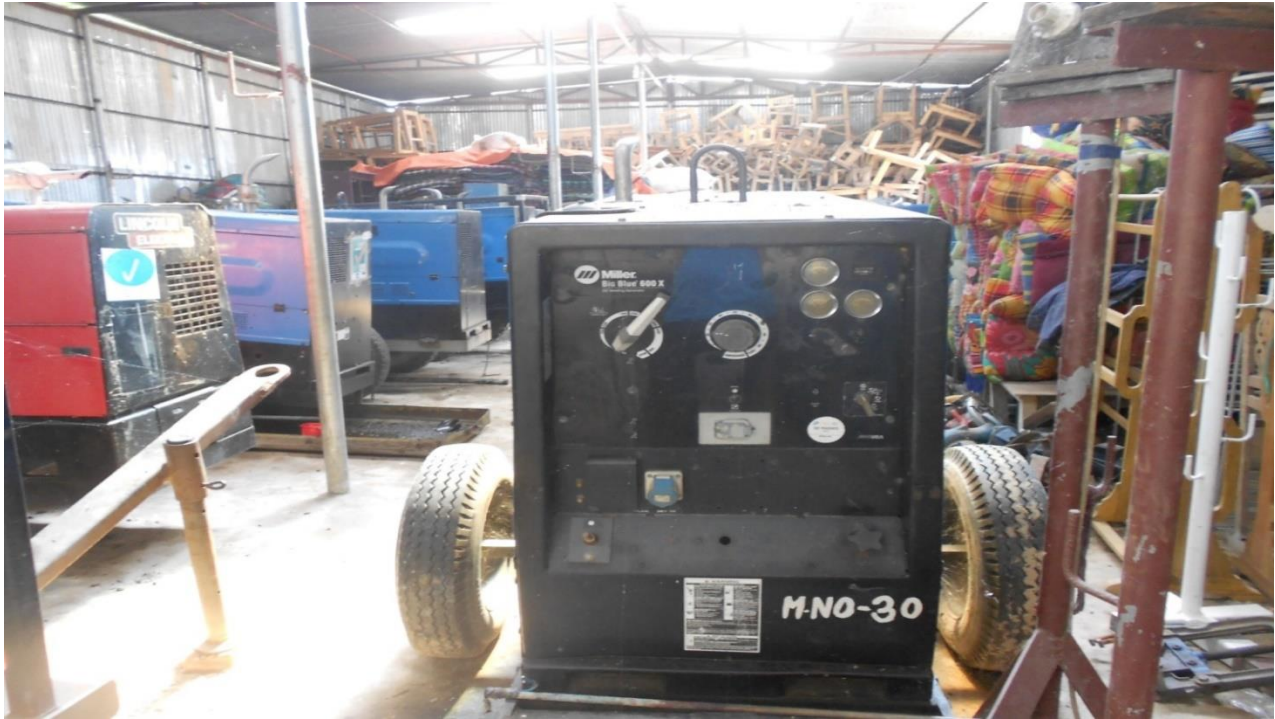
Temporary Equipment and materials Shed
